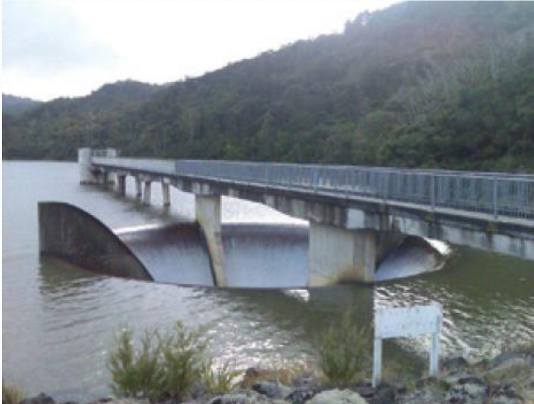
Bellmouth and tunnel spillway
